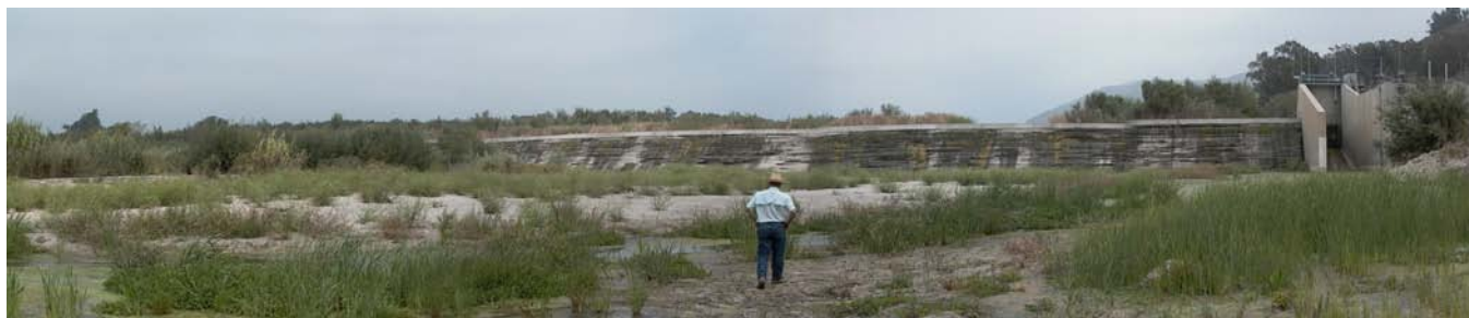
Looking upstream to Vern Freeman Diversion Dam (2003). (photograph by Stillwater Sciences)
