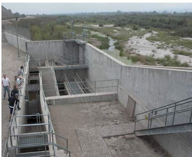
(top) Looking upstream, and (bottom) downstream at the at the Vern Freeman Diversion Dam fish ladder (2003). (photograph by Stillwater Sciences)
